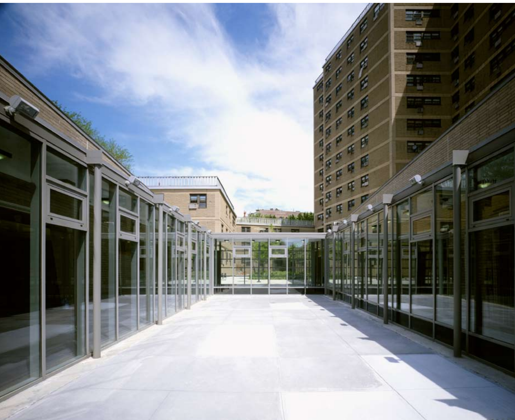
Above: Structure exposed within courtyard; Below: Building courtyard
